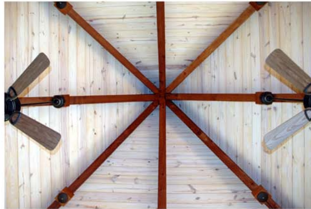
Cedar Beam, Tounge & Groove Ceiling
